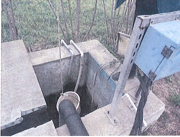
DW001 (厂区总排口)
